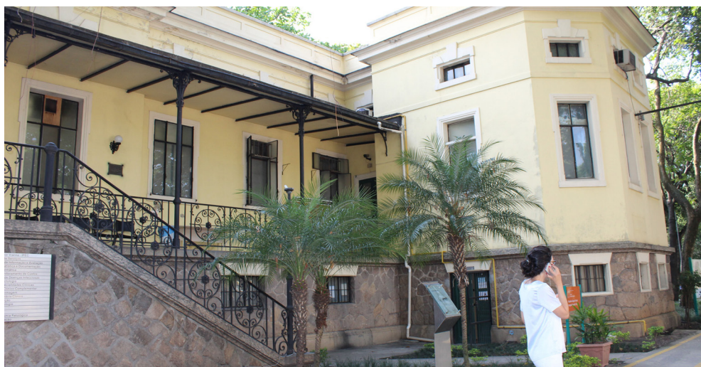
Figura 4. Fachada frontal – Hospital Evandro Chagas – 2017 (DPH/COC/FioCruz).
